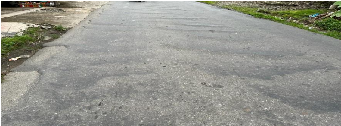
Figure 1. Wavy Damage to Flexible Pavement (Researcher)
